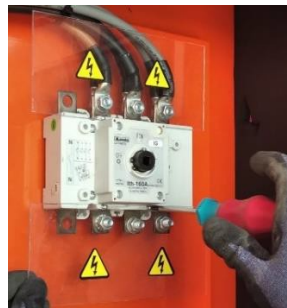
Figure 15: Extraction of safety panel
