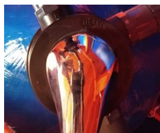
Figure 38: ACF Back-Wash selector
